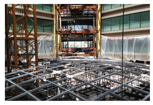
Work is under way to install 404 glass panels on one of the key architectural elements in the new structure—the glass dome in the atrium.
