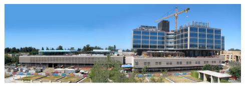
The oversized double-glass wall, which runs from patient levels four through seven, will allow future patients sweeping views of the foothills and surrounding Stanford campus. The clear-vision glass windows include an energy-efficient intelligent shading system with motorized blinds that offers a more sustainable way to control climate inside the hospital.
